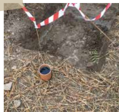
Fig 1c: Soil pipe infiltration test
